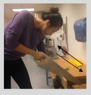
13. Mark a 1" x 1" (2.5cm x 2.5cm) square in the center of the long piece of wood with a pencil. It is useful to mark an "X" on the wood by connecting the corners in order to find the center (where the lines intersect).
