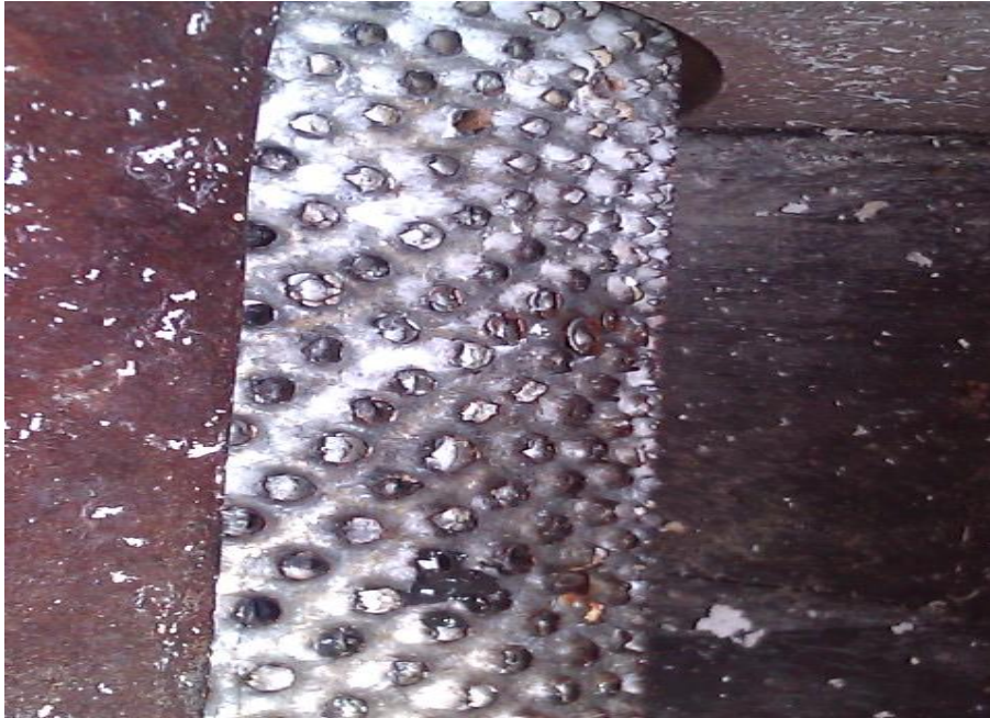
Figure A 1: Grating Surface of Drum at Esuogya site 1
