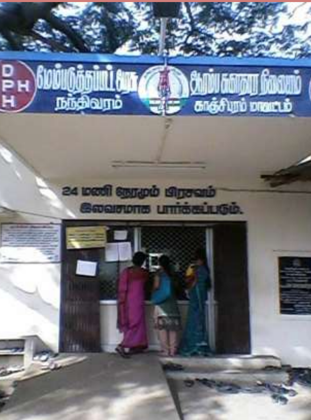
Primary Health Centre (Govt) Guruvancherry (9.8 km)
